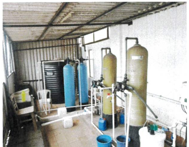
RO Water Plant Installed in the campus
