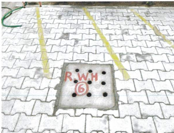
Rain Water Harvesting Soak pit
