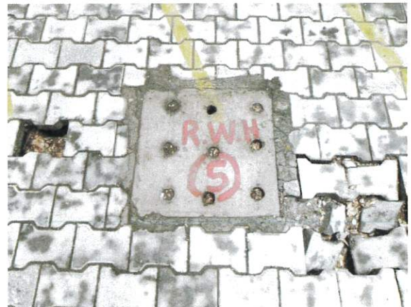
Rain Water Harvesting Soak pit
